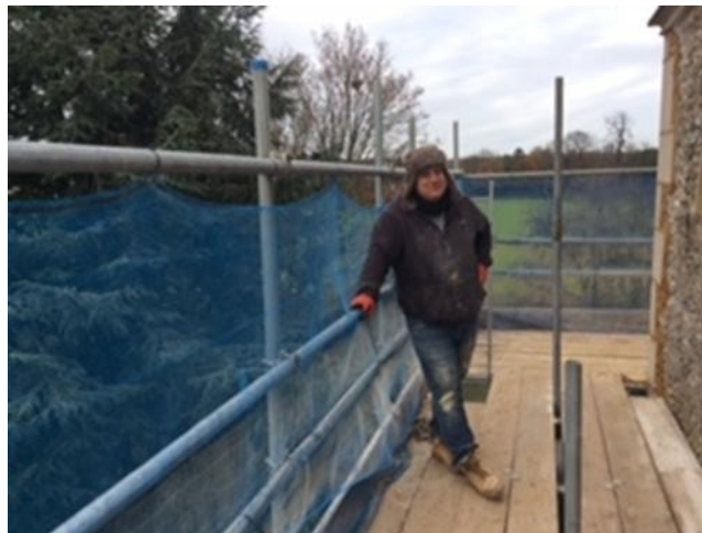
Rob, the head Mason, at the top of the tower
